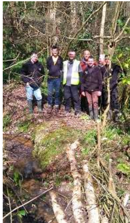
Fig 8. Volunteers installing Leaky Dams at Rivacre Brook
